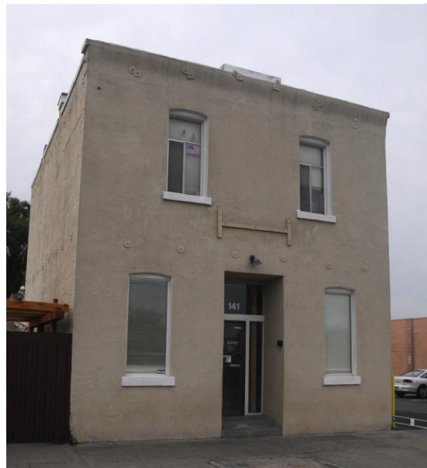
141 Livermore Avenue.* Both buildings were in the Gardemeyer Block.
