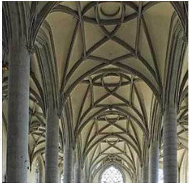
The gothic ribs in the ceiling of St. George Church in Nordlingen, Germany. Treva Mitchell’s sculpture brings to mind this intricate pattern.
